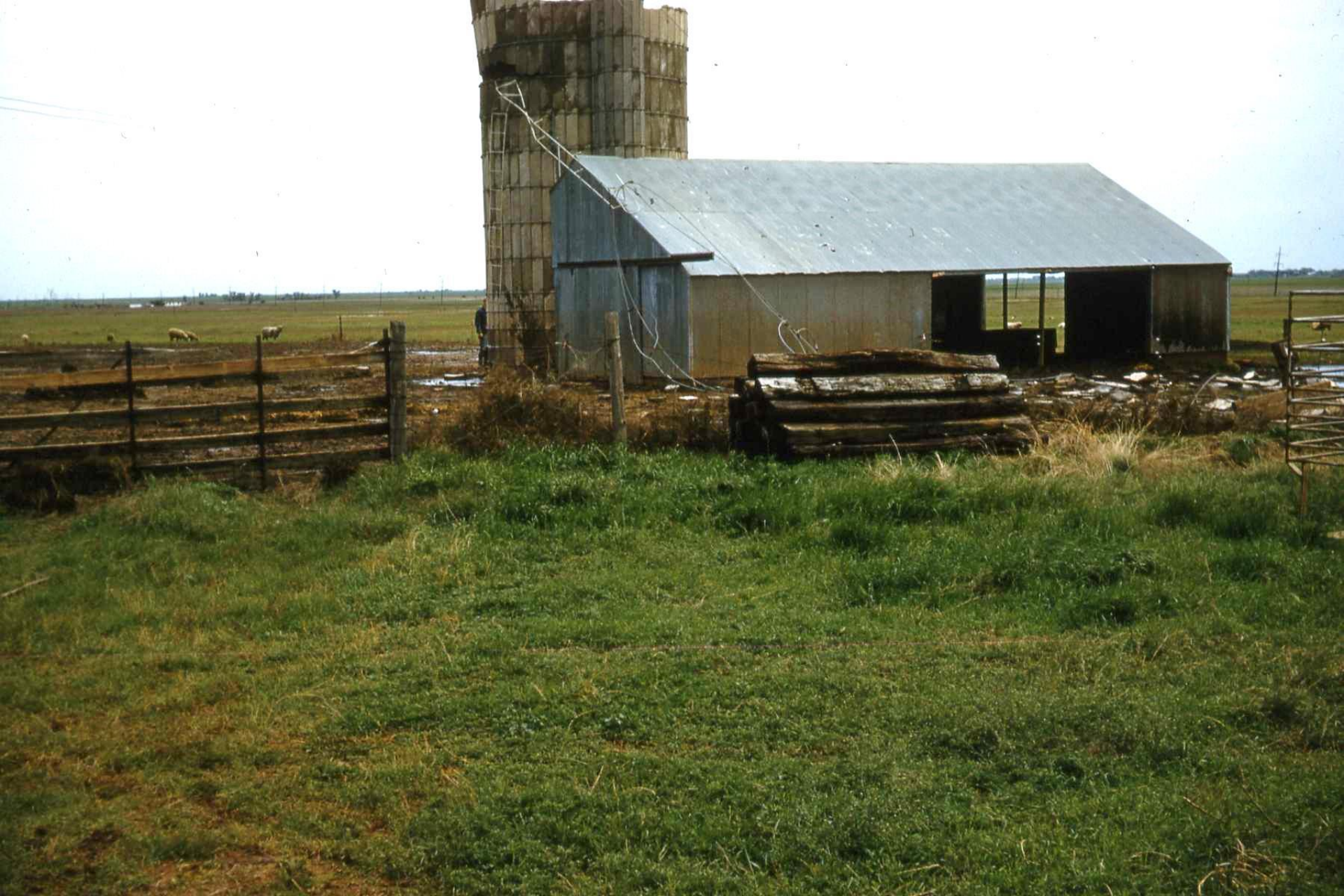
Jake Regier slide: Silo shed & silo, looking NNE - note ladder and top crib railing hanging on roof, silo blocks, & pickup stock rack @ extreme R. Ruben & Sophie Thesman home at back L.
