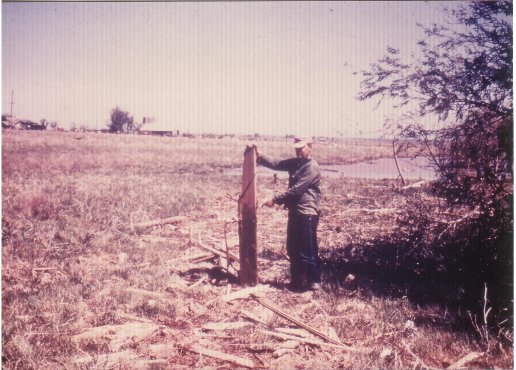
TORNADO0006: Robert P (Bob) Voth in George Ediger's pasture S of our home-place, showing a barn rafter that was driven into the ground ~3 ft by the tornado. There were more than one of these. [Non-adjusted photo of previous slide]
