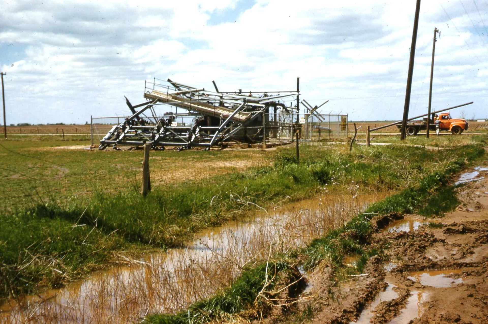
Jake Regier slide: Destroyed OG&E electric substation @ NE corner of 12 Acres, looking NNW from Wall Street. OG&E truck on Kremlin Blacktop @ R back
