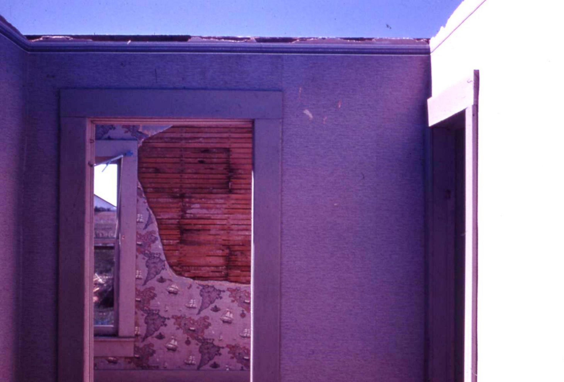
DAT 11-18: Upstairs after the tornado - Toews Brother's bedroom door @ L, Mom & Dad's bedroom door @ R. Note wallpaper and plaster laths in the boy's bedroom, and Carolina Blue sky @top center.
