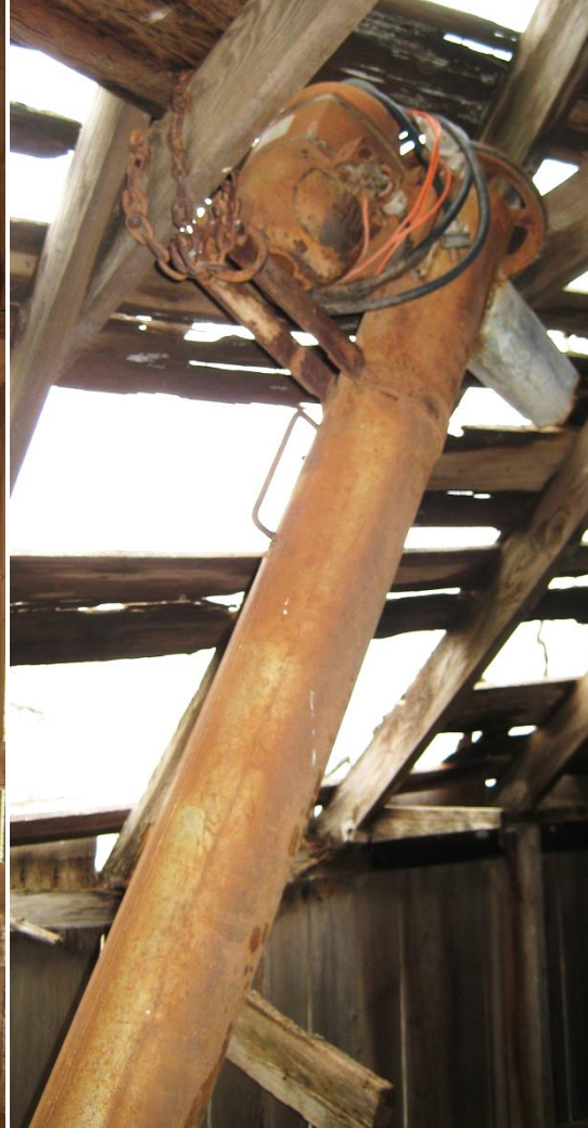
Grain auger suspended on shed rafter
