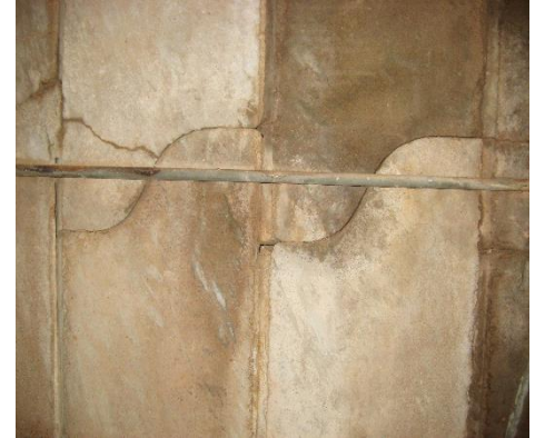
Detail of interlocking silo blocks with metal band
