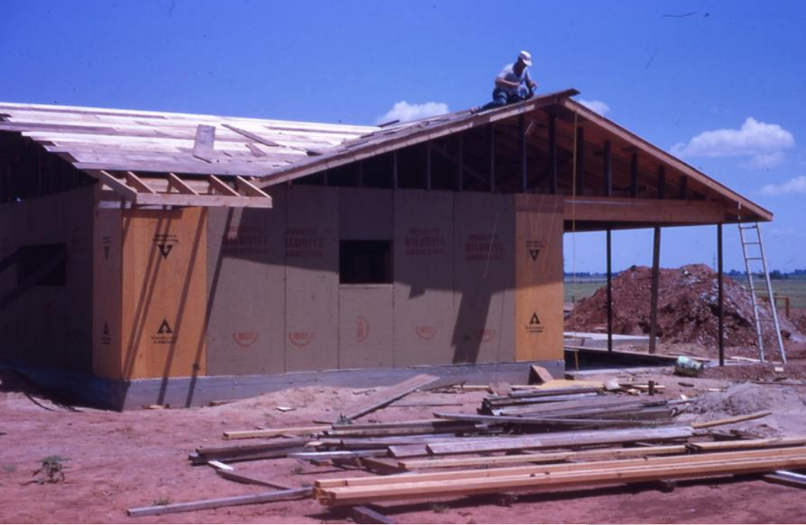
New DAT/RMT house along Kremlin blacktop under construction (1961-62)
